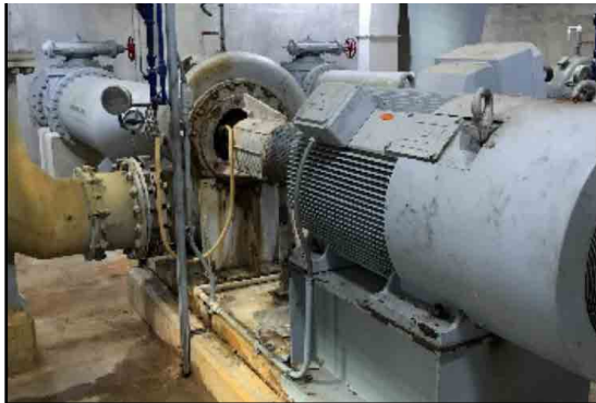
ITT 12 x 12 x 15 NSY End Suction Pump
