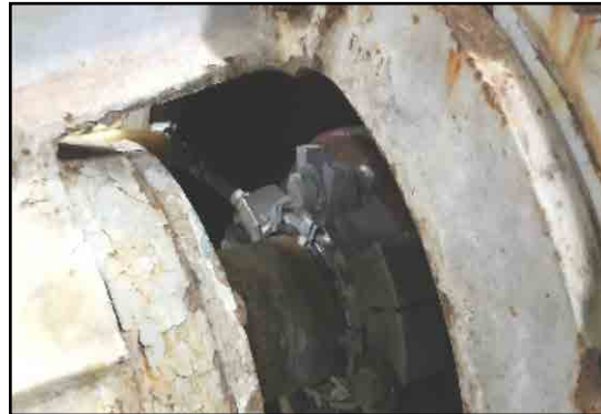
442C Seal 114 mm (4.50") was installed in less than two hours
